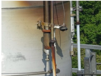
View of Pilot Gas Mixer #3 (225 Degrees) (4" Pilot on the left of the ladder)
