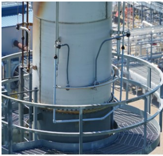
Pilot #1 and #2 Manifold/Conduit
