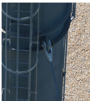
Guy Wire Stack Connection #1 (90 Degrees) (Closest to Ladder)
